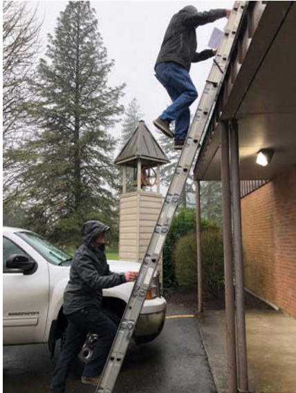
Contractors Pre-Bid Meeting Site Walk
