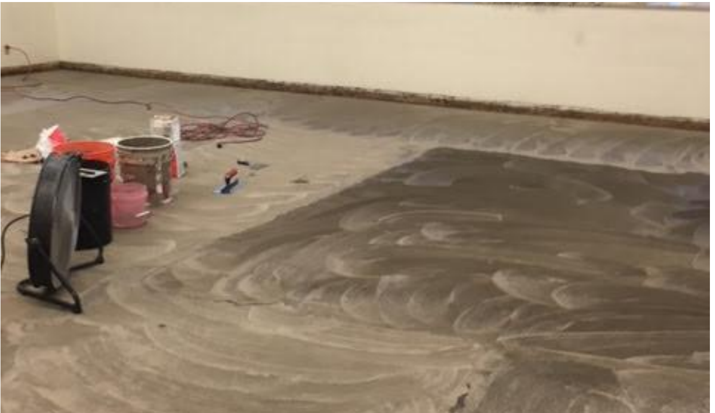
Classroom Asbestos Flooring removal and replace
