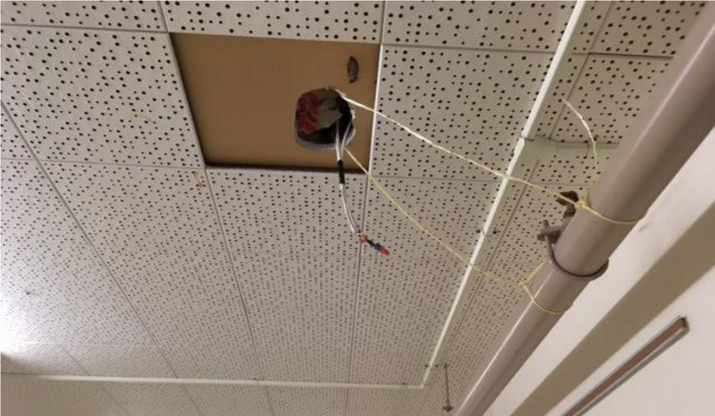
Wires Routed Thru the Ceiling To Minimize The Amount Of Surface Mounted Wire Moulding
