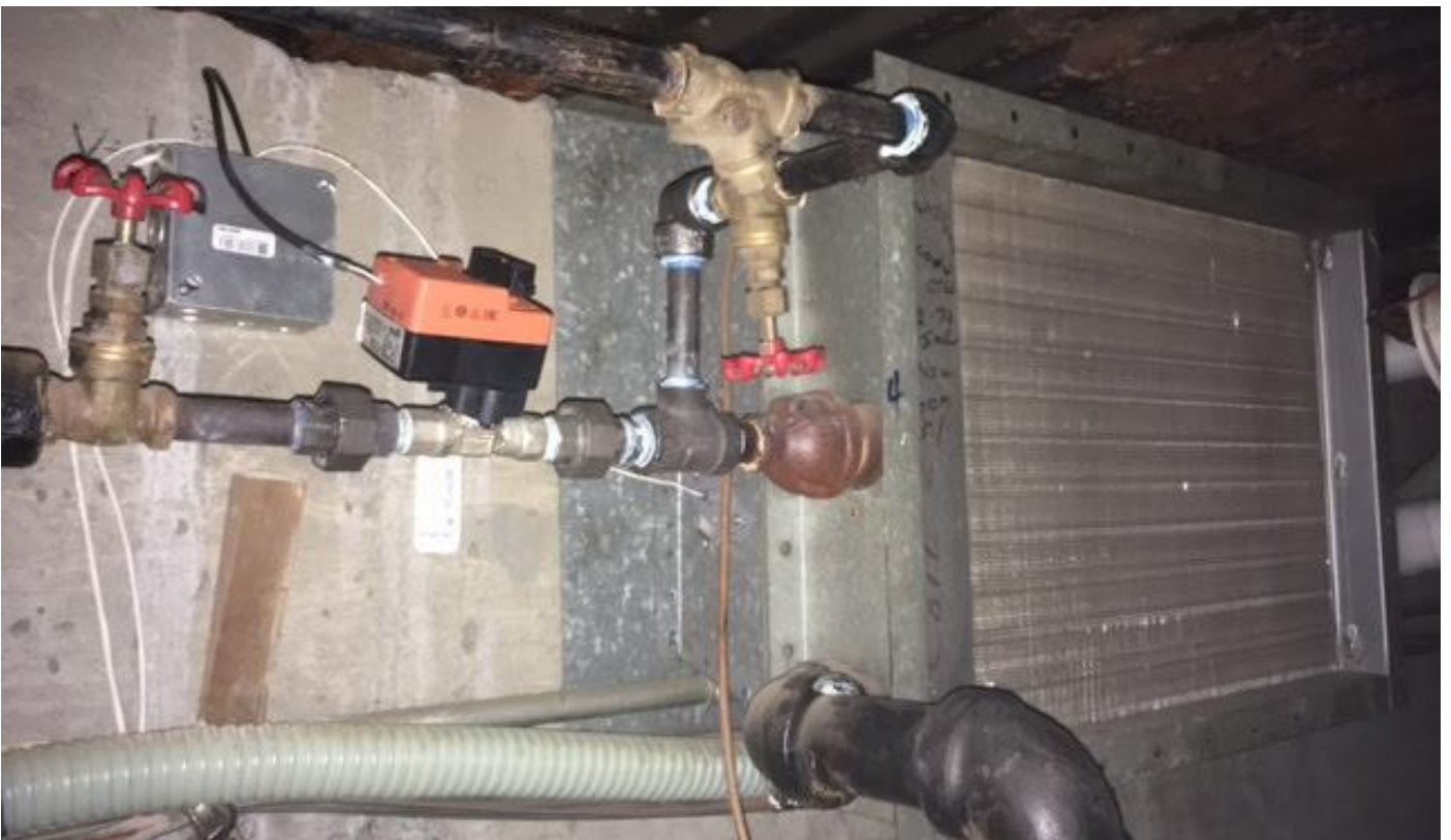
New Valve Installed
