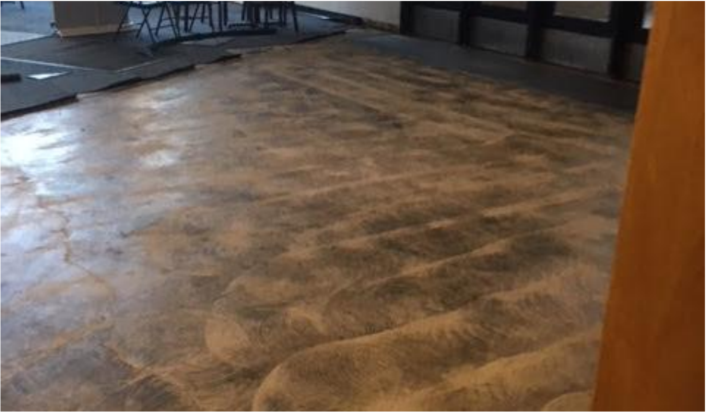
Classroom Asbestos Flooring removal and replace
