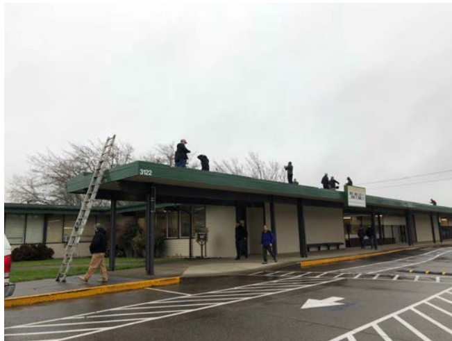
Contractors Pre-Bid Meeting Site Walk
