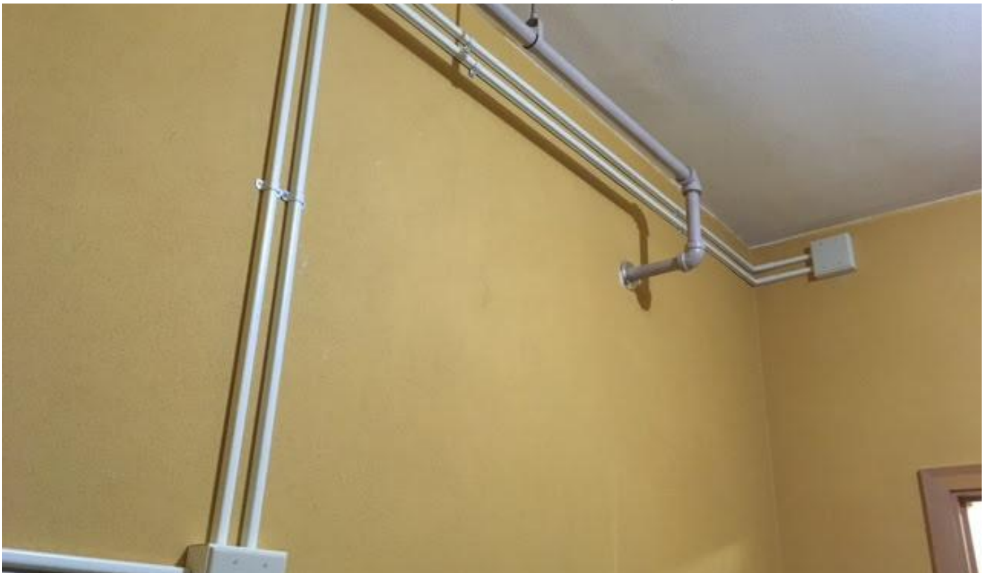
Example of Surface Mounted Raceway
