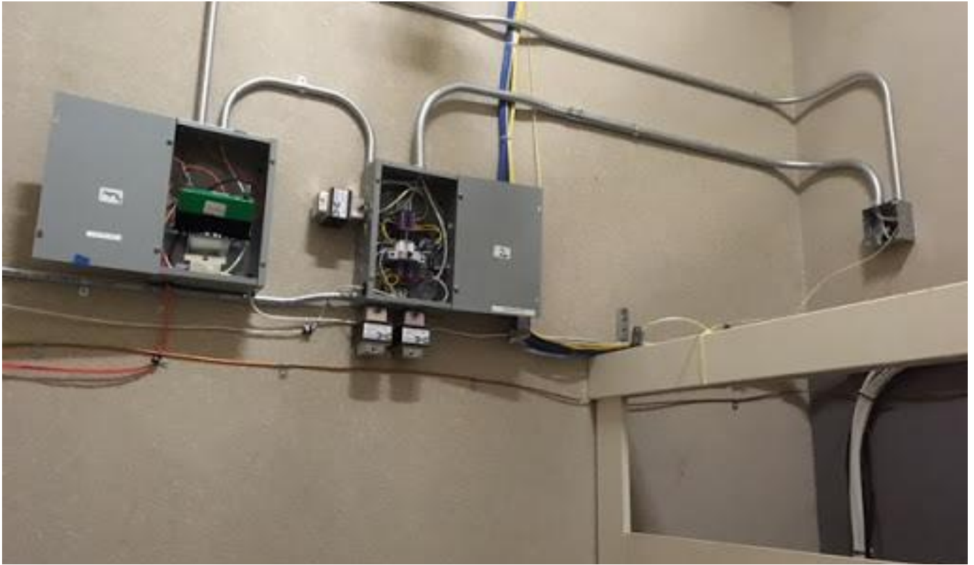
Example of Surface Mounted Raceway
