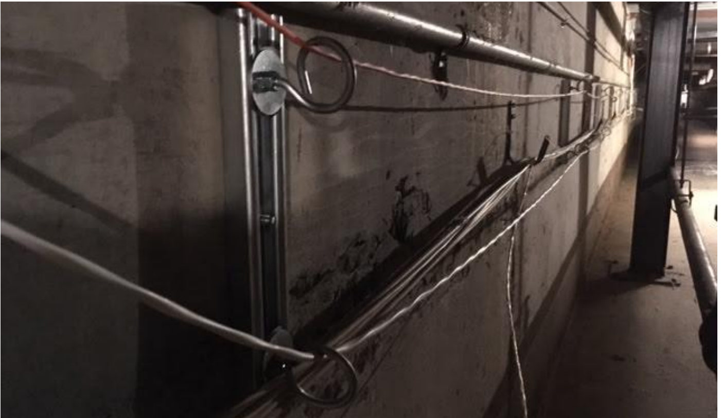
Communication Cable Routed Down Thru The Tunnel
