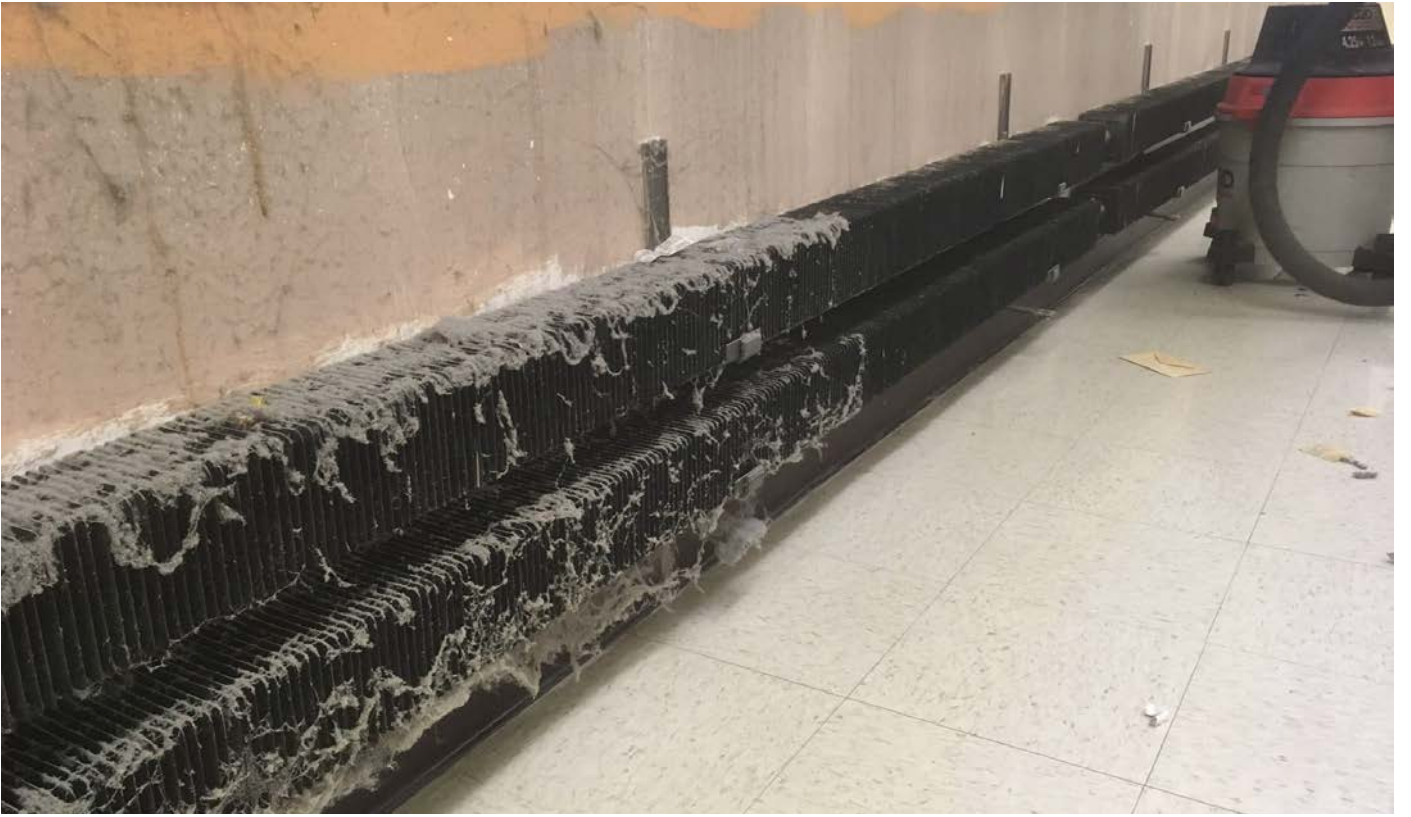
All Coils Cleaned During Winter Break
