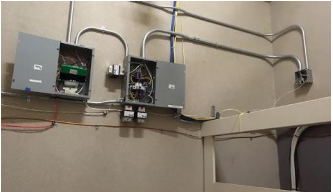
Router And Power Supplies Installed
