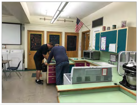
Subcontractor walk throughs to prepare for construction. Food Science plumbing.
