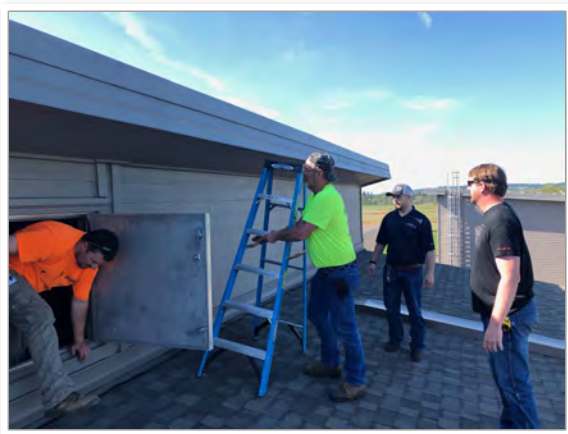
Contractors reviewing preexisting conditions
