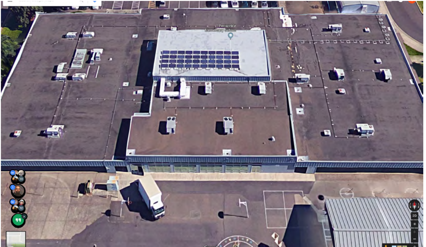
These are the Rooftop units that will be replaced
