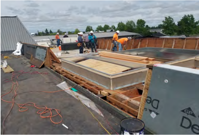
New mechanical equipment curbs being installed.
