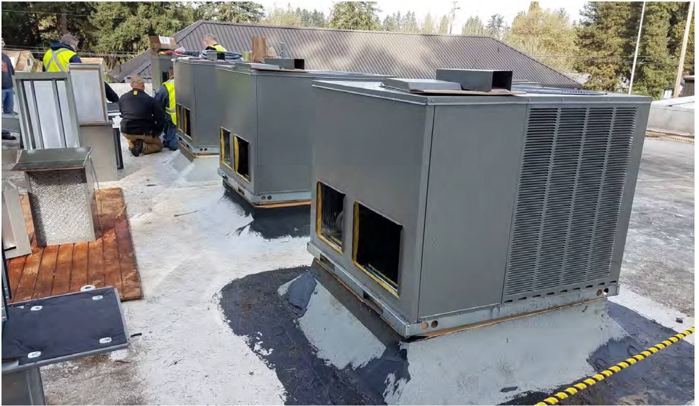
New units placed on roof curbs
