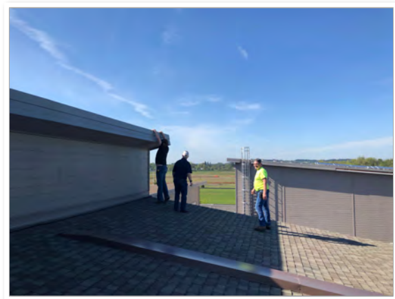
Contractors reviewing preexisting conditions
