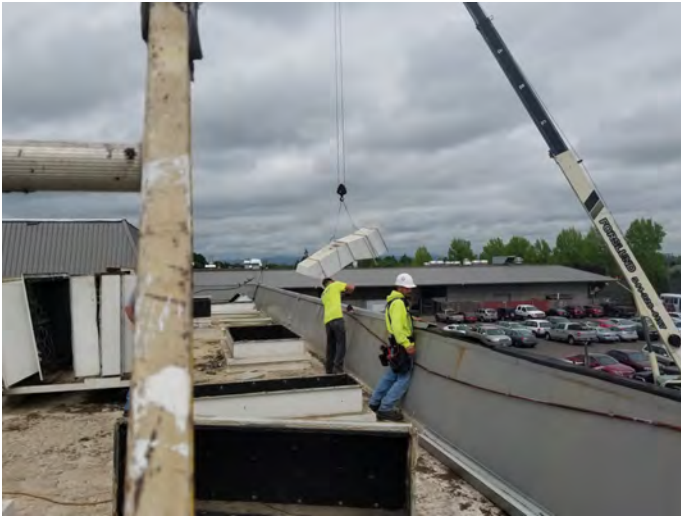
Portions being lifted off.
