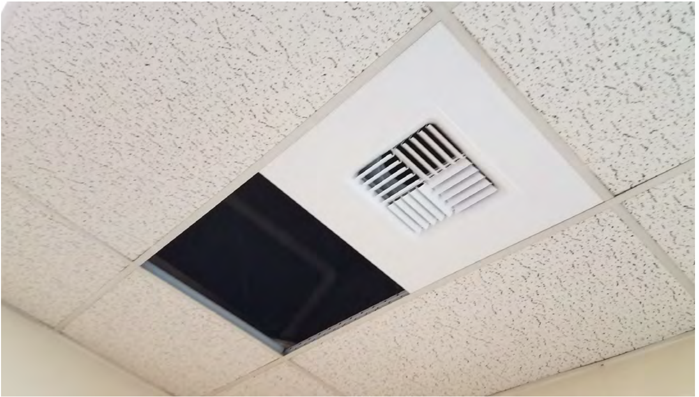
New supply grills being installed in the ceiling
