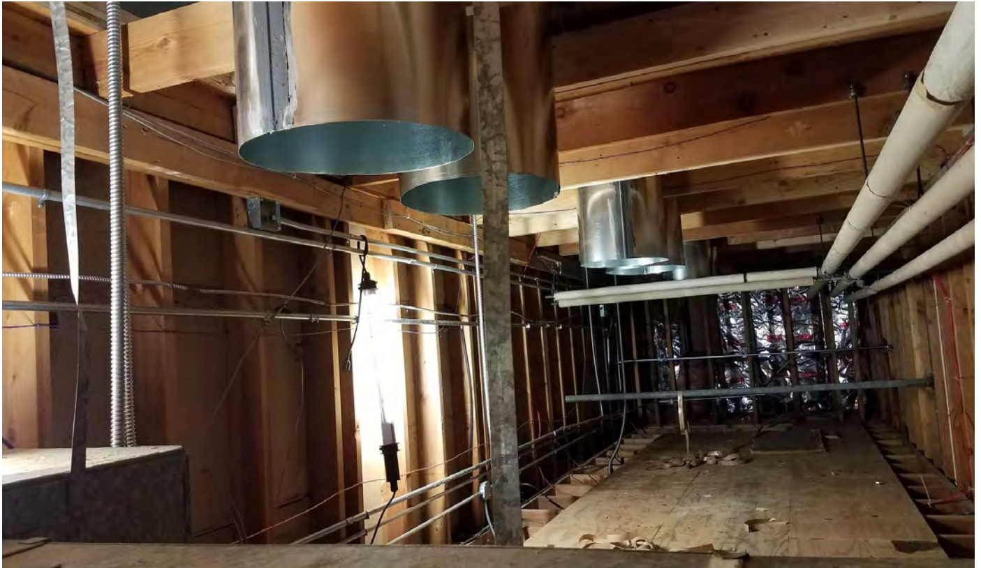
These are the drops from the units for the new ductwork to attach to
