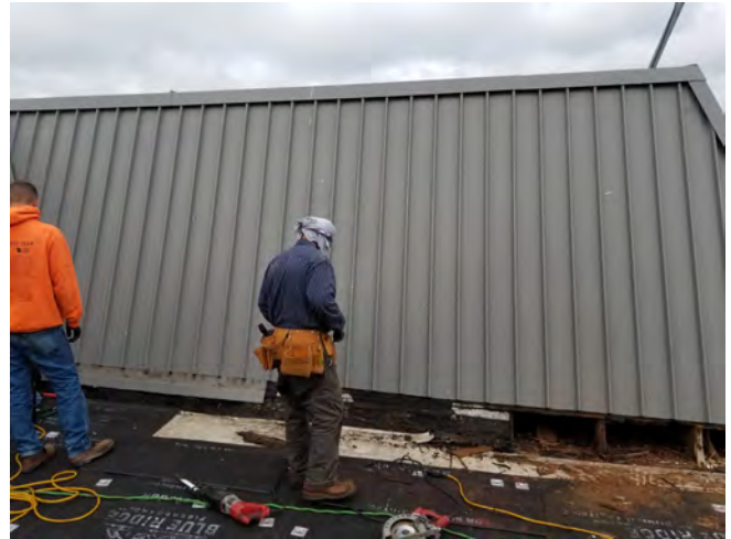
Pool Building. East side front parapet wall. Underlayment for wall rotted. Metal to be removed/reinstalled and plywood replaced.
