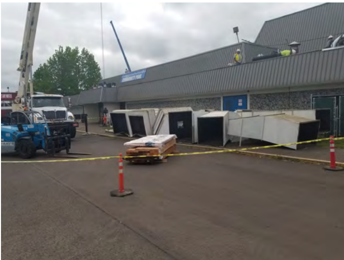
Old equipment awaiting disposal.
