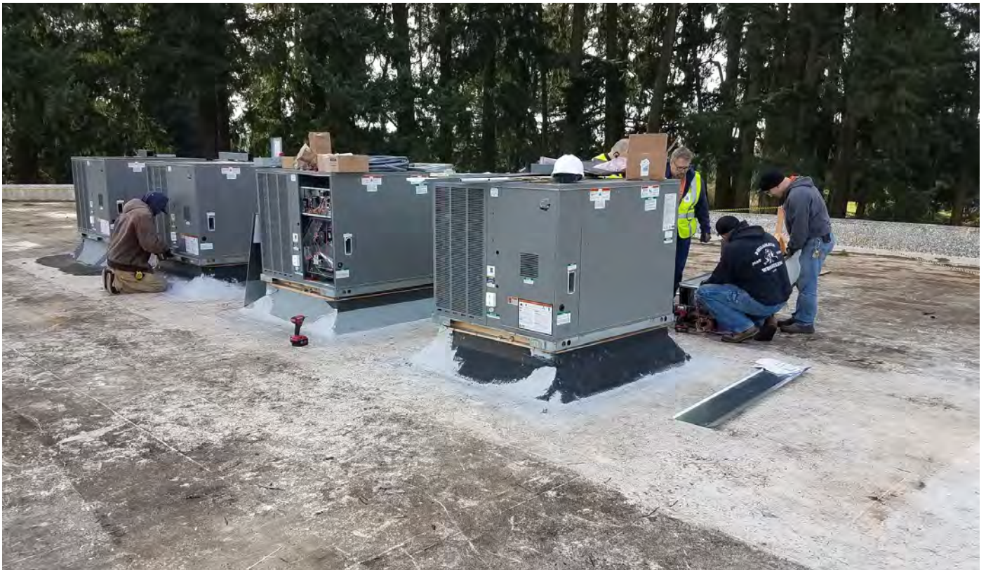
These four units replace the old 100% electric classroom ventilators with gas Rooftop Units
