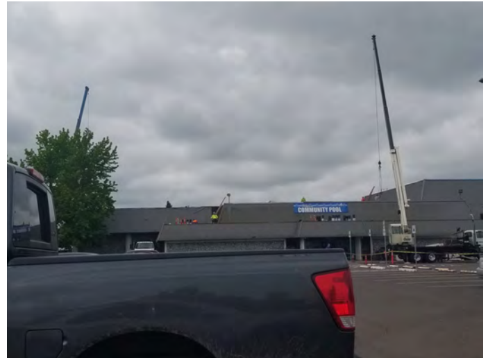
Roofing and mechanical projects working together both with cranes onsite.
