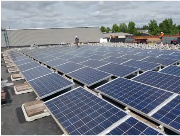
Solar panels being reinstalled
