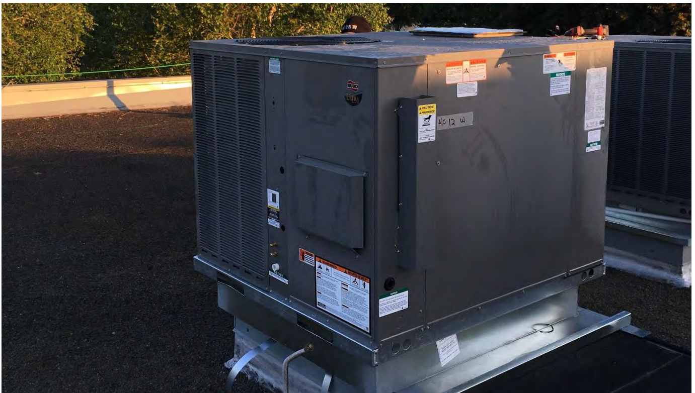
New unit installed
