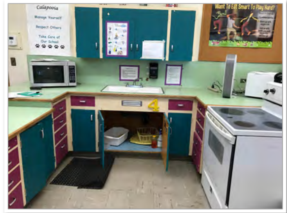
Subcontractor walk throughs to prepare for construction. Food Science plumbing.
