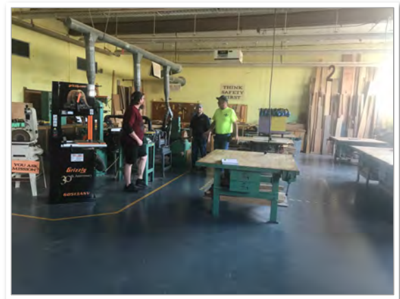
Wood Shop sheet metal for new dust collection system.
