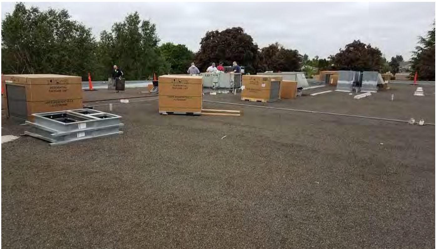
Units lifted onto the roof ready to install
