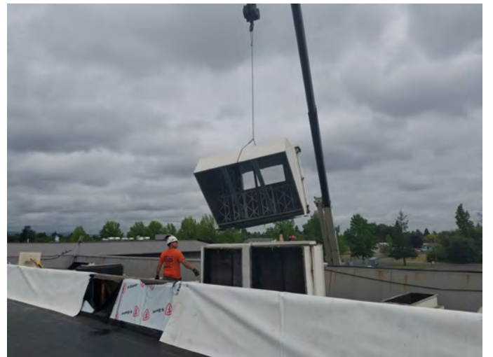
More equipment removal.
