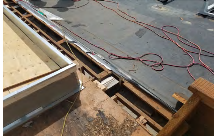
New steel structural beam installed to support new mechanical equipment
