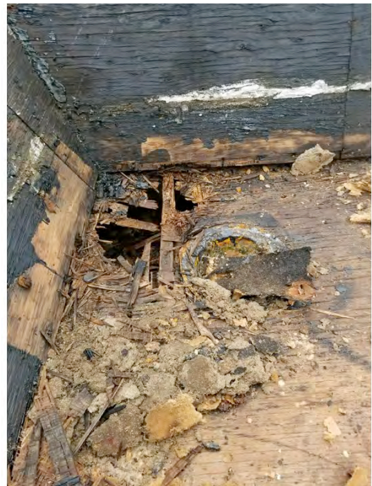
Pool Building. North East front corner drain. Plywood and new drain to be installed.
