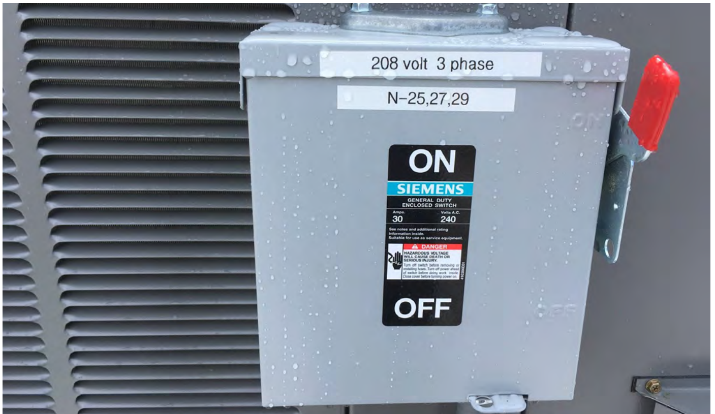
New electrical disconnect for each unit
