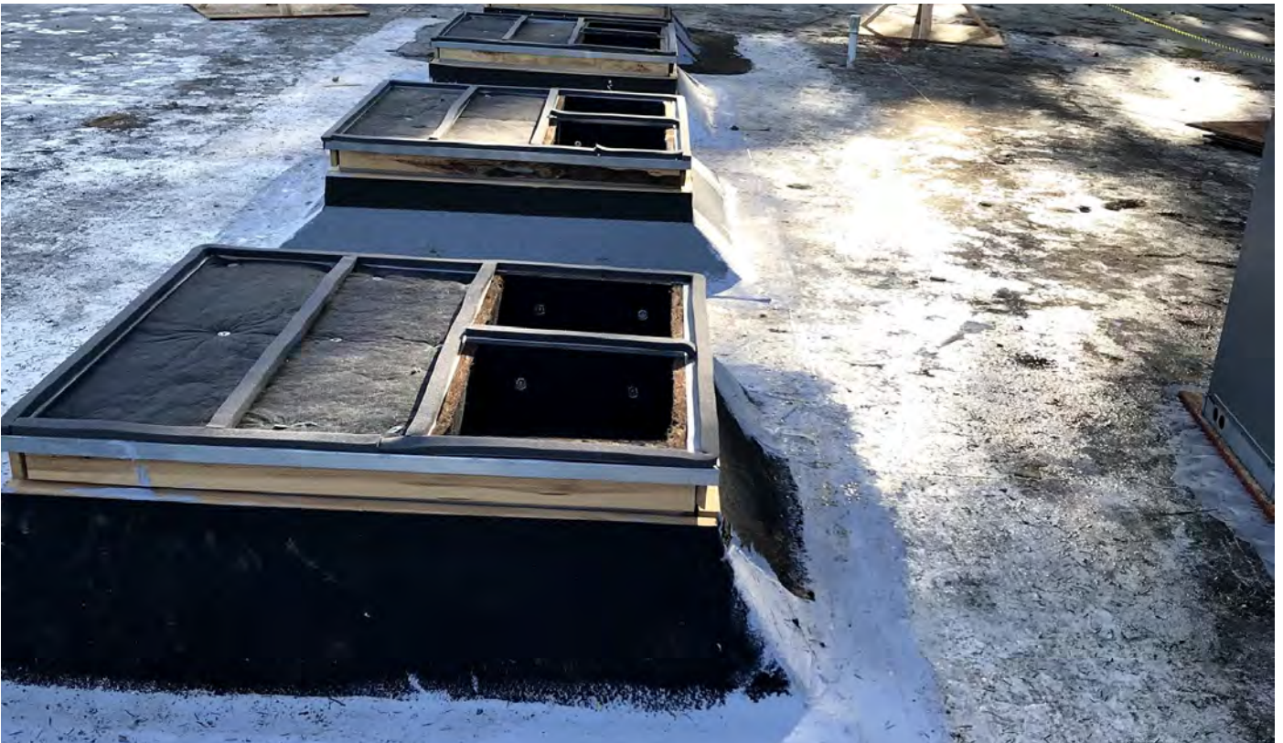
New roof penetrations to install new roof top units
