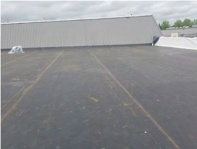
Pool Building. Main roof nearing completion. Upper roof in background having metal trim installed
