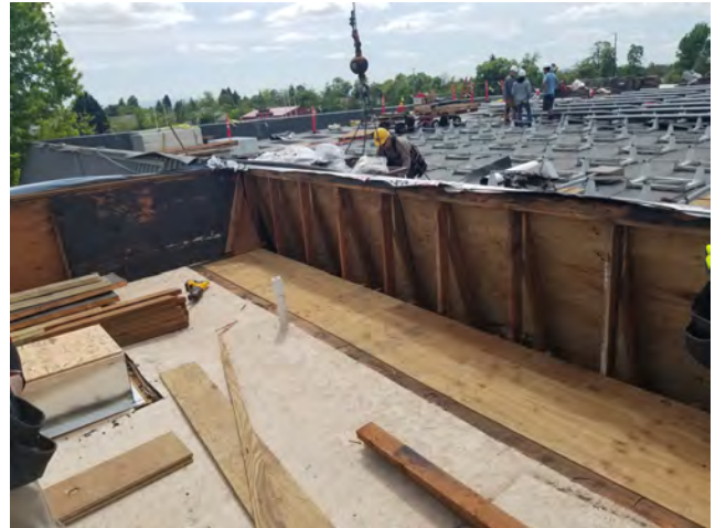
Parapet wall and outer edge of decking lumber replacement
