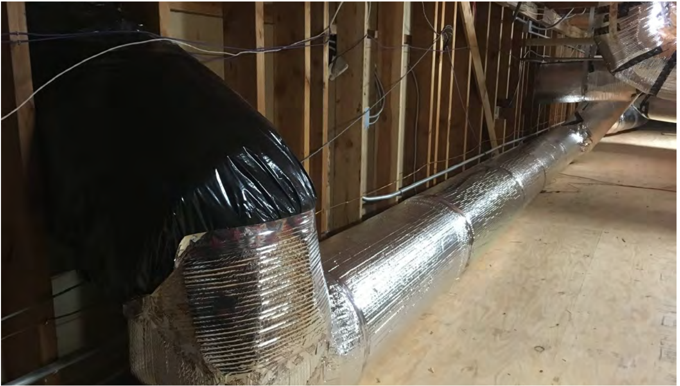
New Duct Work
