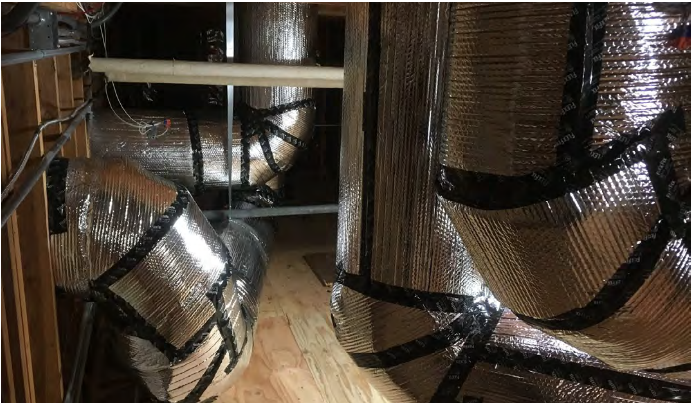
New ductwork to new rooftop unit
