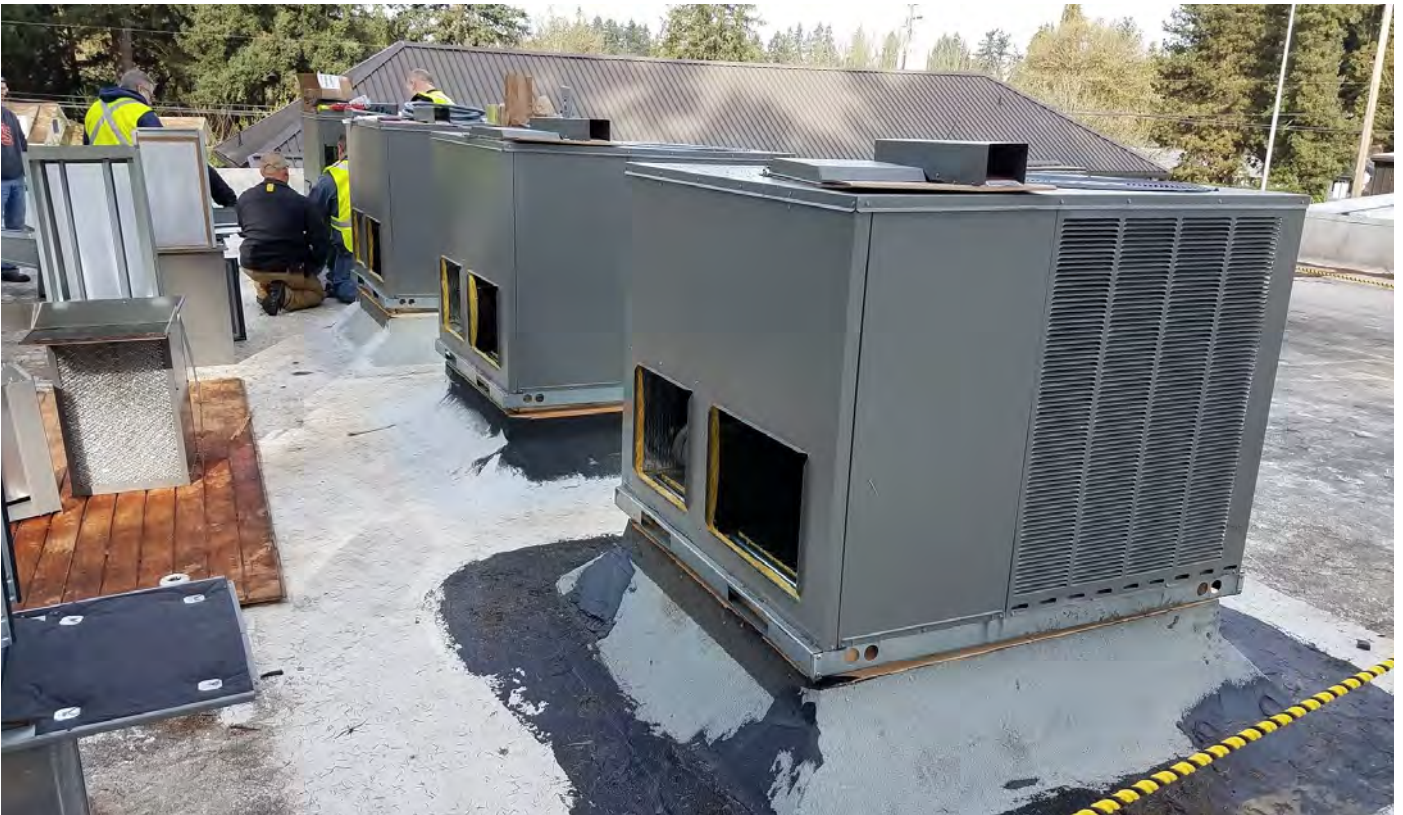
New units placed on roof curbs
