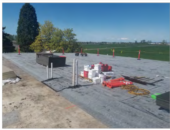
Day two Northwest view with new base layer of roof in place at Facilities.
