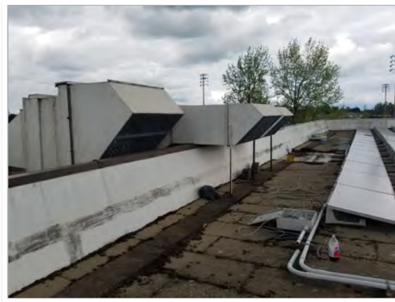
Existing equipment on roof to be removed. A section of the parapet wall below to be lowered to install new equipment
