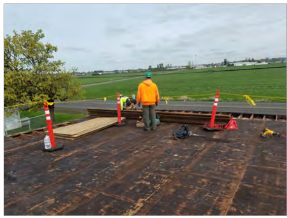
Photo of perimeter lumber being replaced at Facilities.
