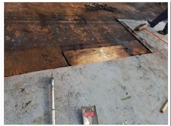
Photo of the past under the roofing. Several skylights had been removed and roofed over at Facilities.
