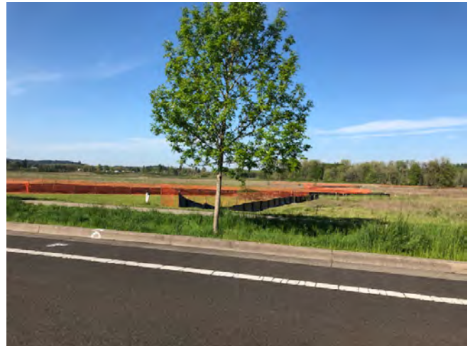
Erosion control: silt fence and snow fence have been installed at the new Meadow Ridge Elementary School site.
