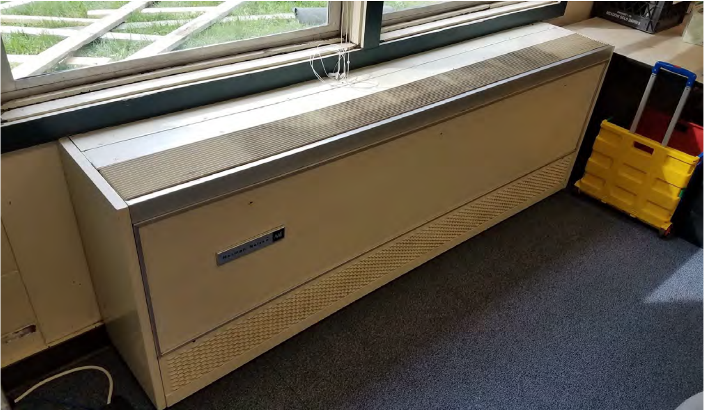
Old classroom ventilators to be removed after the new units are up and running
