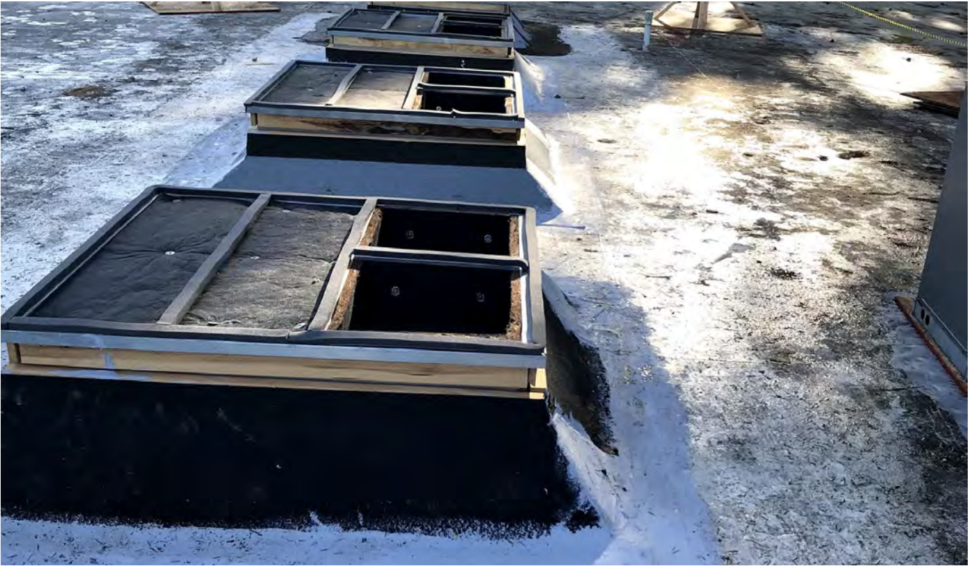
New units placed on roof curbs
