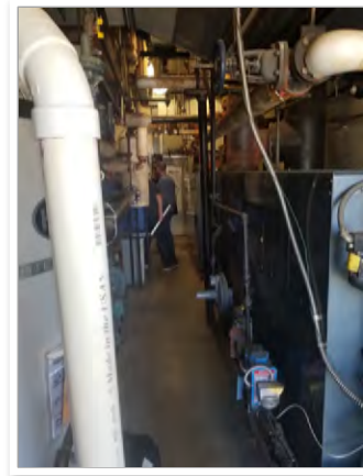
Electrical and mechanical contractor coordination.
